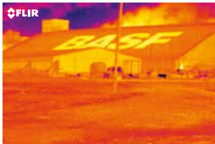
BASF has been using thermal imaging cameras for a long time.
