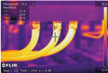
Thermal image of electrical cables.
