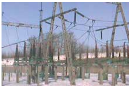
150 KV station, visual and thermal images.
