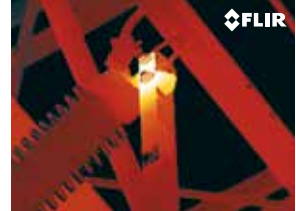
Incorrectly secured connection
