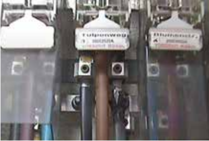
This connector has become resistive due to loosening and corrosion. This can be easily remedied by opening, cleaning and reassembling the connector.
