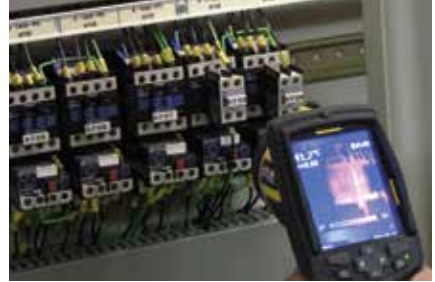
Inspection of a fuses in an electrical cabinet.
