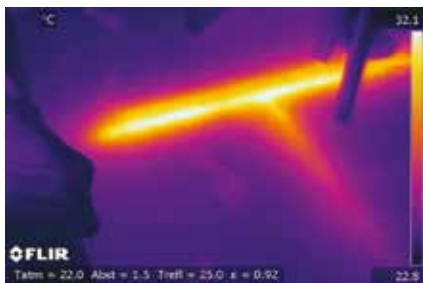
This thermal image shows where the hot water pipe has been installed beneath the floor.
