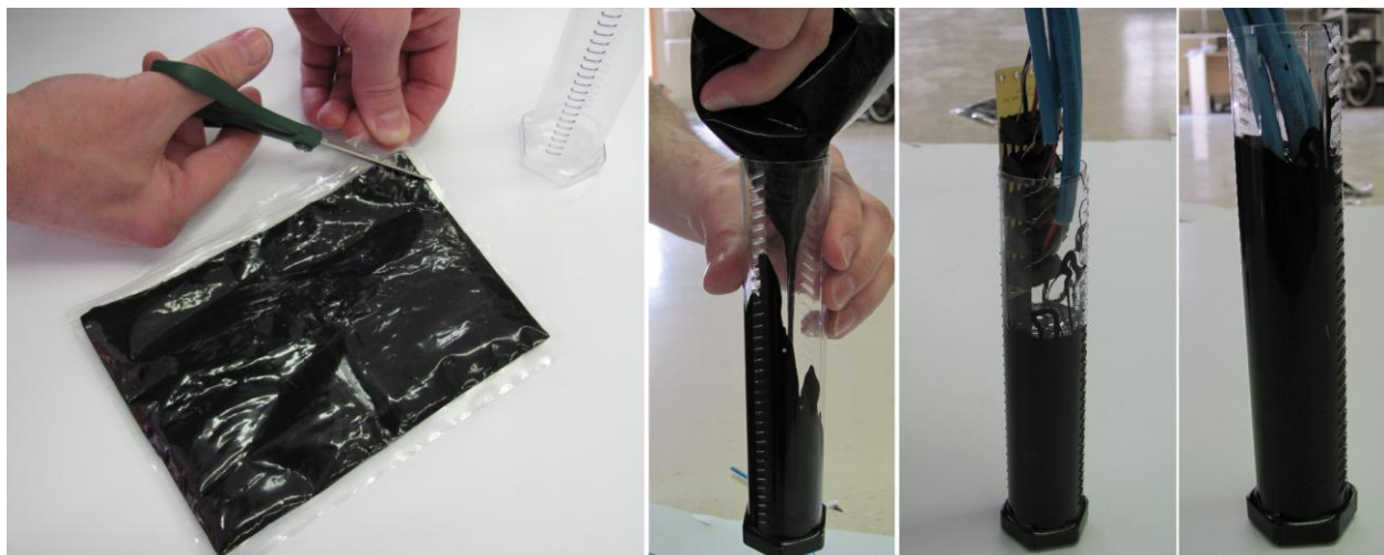
Figure 4.6: Potting SAATERM with SAA and SAAPZ cables spliced together.
