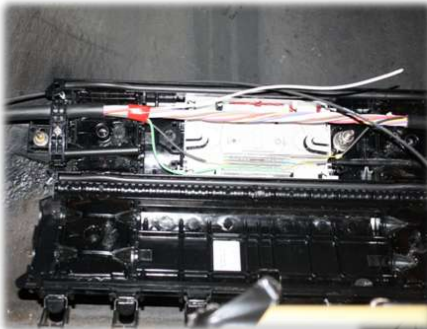
Tapping into the main cable feed at various locations along the bridge. (above)
