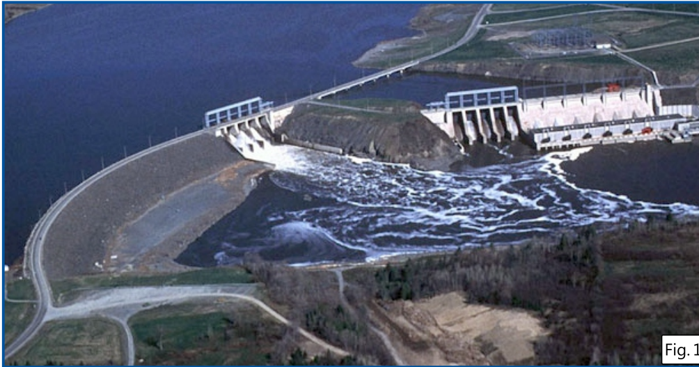
Figure 1.: Mactaquac Dam, located in Keswick Ridge, NB.
