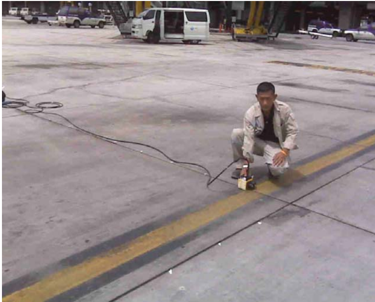
Tests site in the International Airport of Bangkok
