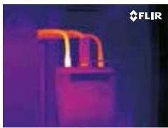
Poor connection and internal damage
