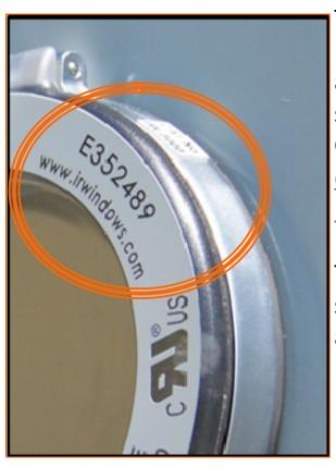
The IR Window shown here displays the E Number which engineers can use to access further information on the specific IR Window from the UL Online Certification Directory, <a href="http://database.ul.com/cgi-bin/XYV/template/LISEXT/1FRAME/index.htm">http://database.ul.com/cgi-bin/XYV/template/LISEXT/1FRAME/index.htm</a>
