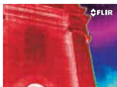
Thermal imaging reveals a hidden window construction invisible to the human eye.
