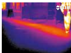
Leaks in an underground district heating network.
