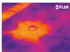
The thermal image shows water leakage in the roof.
