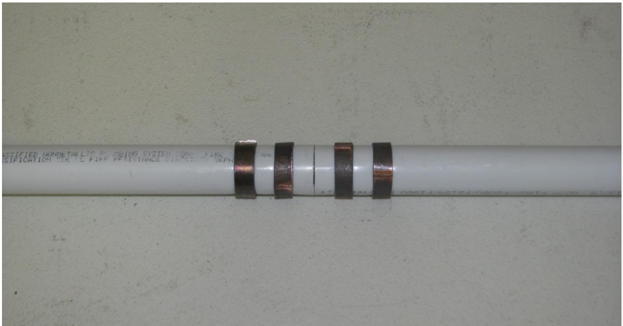
Figure 3.4 – Step 4. Repeat Steps 2 and 3 for other side of PEX connection. The final result should resemble the assembly shown above.
