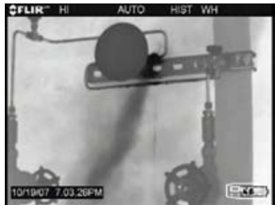
A leaking pressure gauge
